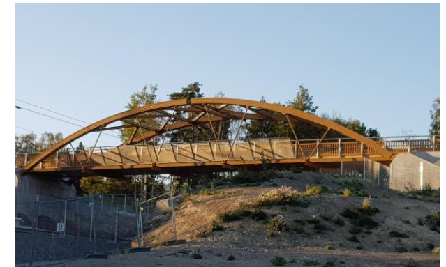
Vega footbridge at Haninge.
